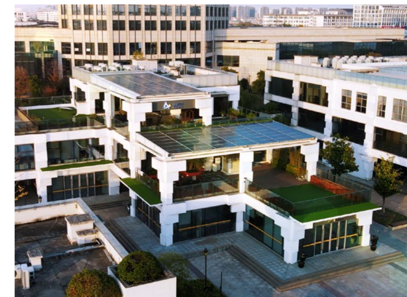
Roof photovoltaic project of AlphaESS Suzhou Branch
